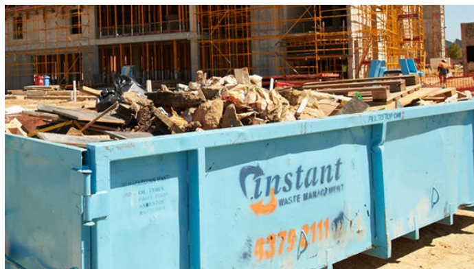
5. Skip bins must be utilised during construction
