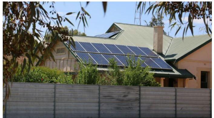
21. Solar panels and other infrastructure should not be visible from the street
